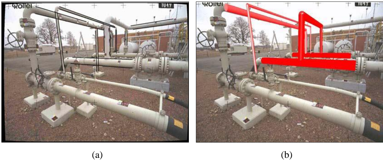
Fig. 5. (a) An images of a part of an oil refinery. The occluding edges of nine straight pipelines are marked in the image. These edges are used to estimate the relative orientation of the image.
