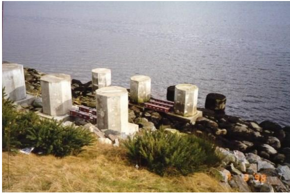
Fig. 14 - Shows the location of the pier stem (right hand side of the picture) near the Dornoch bridge, Scotland
